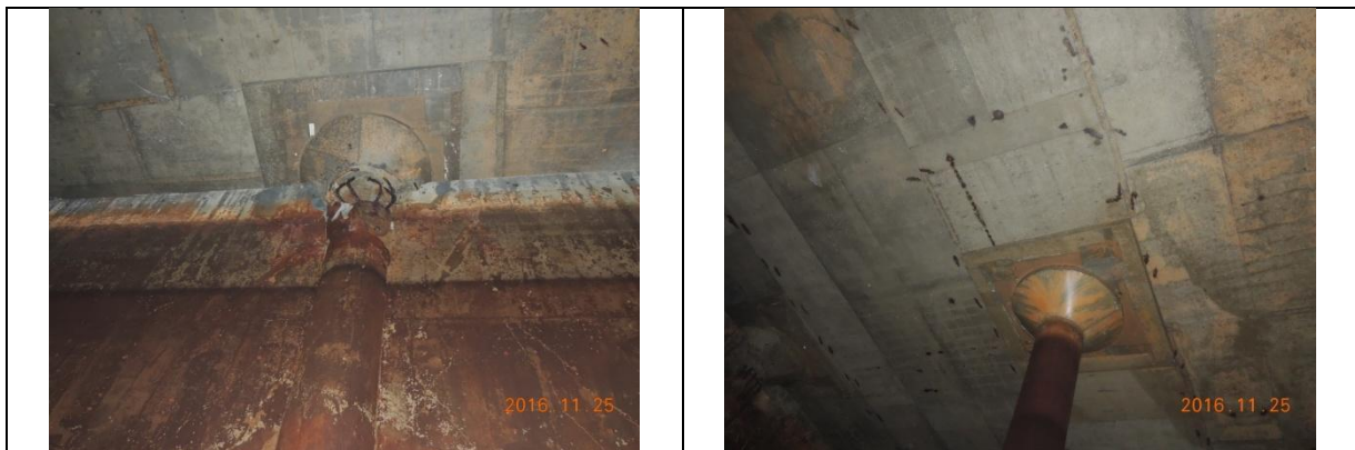
Figure 4. Exposure of Reinforcing Bars Within Columns of Nangang Distribution Reservoir
