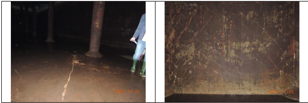
Figure 3. Damages of Nangang Distribution Reservoir by On-Site Inspection
